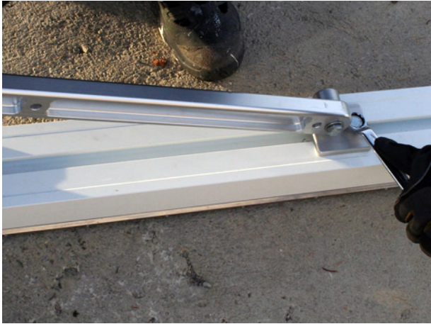
d. Tighten the upper bolt loosely.
