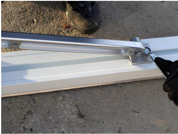
d. Tighten the upper bolt loosely.
