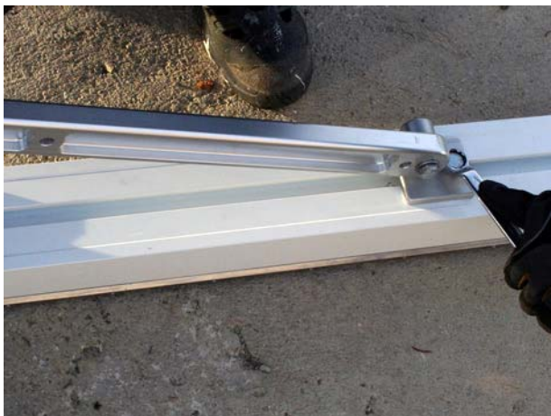
d. Tighten the upper bolt loosely.
